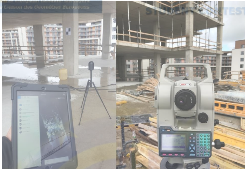
1. Figure, Construction site measurements using TPS and Laser Scanner (Author)
